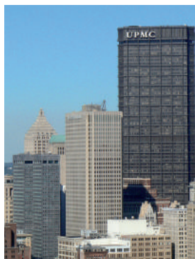
US Steel Tower, 217 mètres Pittsburgh, PA, 1970 Harrison Abramovitz and Abbe architectes
