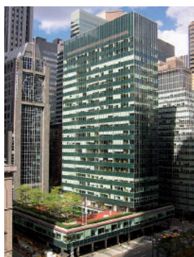
Lever House, 94 mètres New-York City, NY, 1952 Skidmore, Owings and Merrill Gordon Bunshaft architectes
