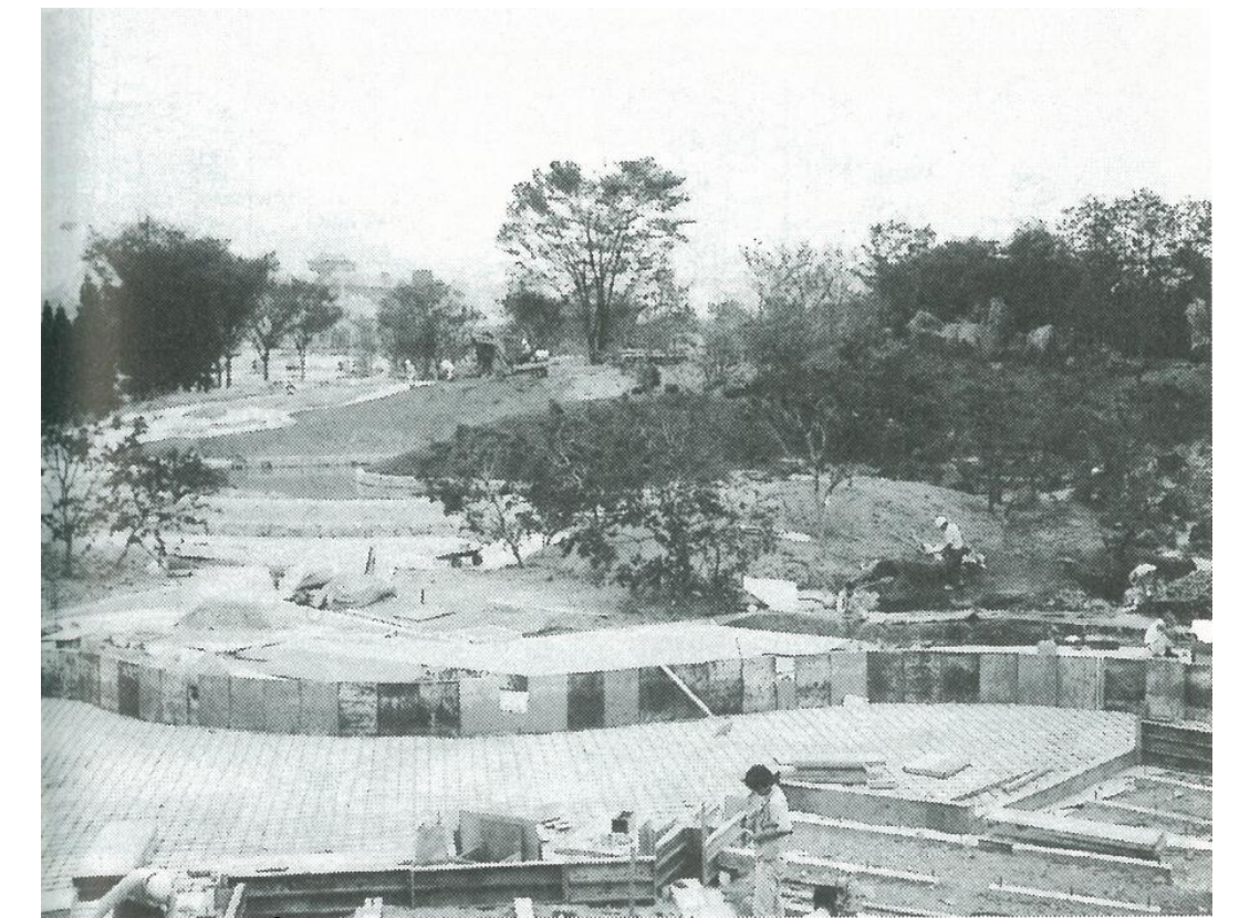
7. Overview of the pool in construction
