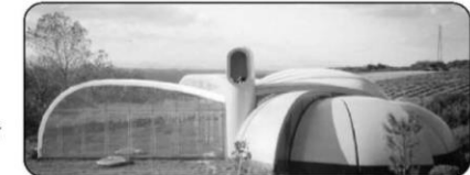
Figure 33. Hulls molded by glass reinforced resin _home of Martine and Pierre Jovine Colleu. (Habitat n°25)
