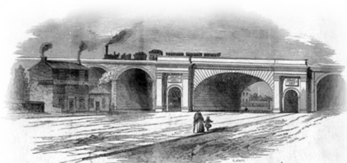
[WICKER VIADUCT, SHEFFIELD.]
