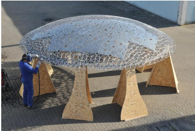
Figure 13: Prototype in progress.
